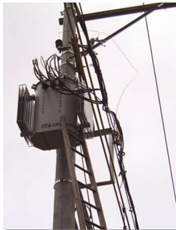
Transformer being installed in pilot area
