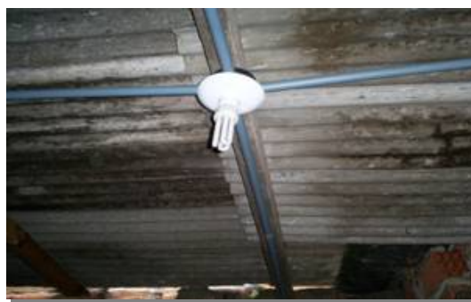
Example of upgraded wiring
